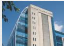
PARAS TWIN TOWERS
